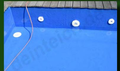
For the renovation of the GRP tile pool, the [DeinTeich.de premium Set](#) with epoxy resin was used for the primer and top coat.
